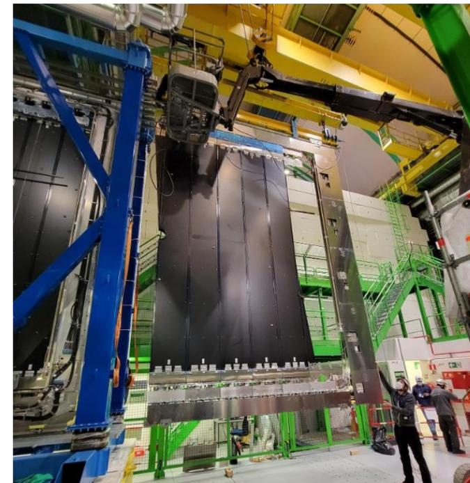
LHCb SciFi C-Frame being installed in the LHCb cavern
