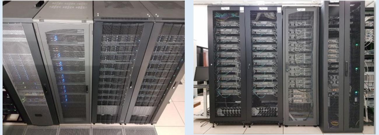
Front view (left image) and rear view (right image) of ARTEMISA racks. Those on the right (left) in the front (rear) view contain the GPU units.
